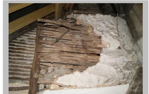
The recent renovation of the attic revealed some of the original features such as the lath and plaster work.
